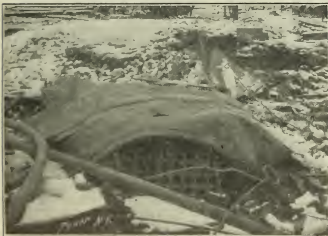
FIG. 3. FRONT HEAD AND BOTTOM OF BOILER
